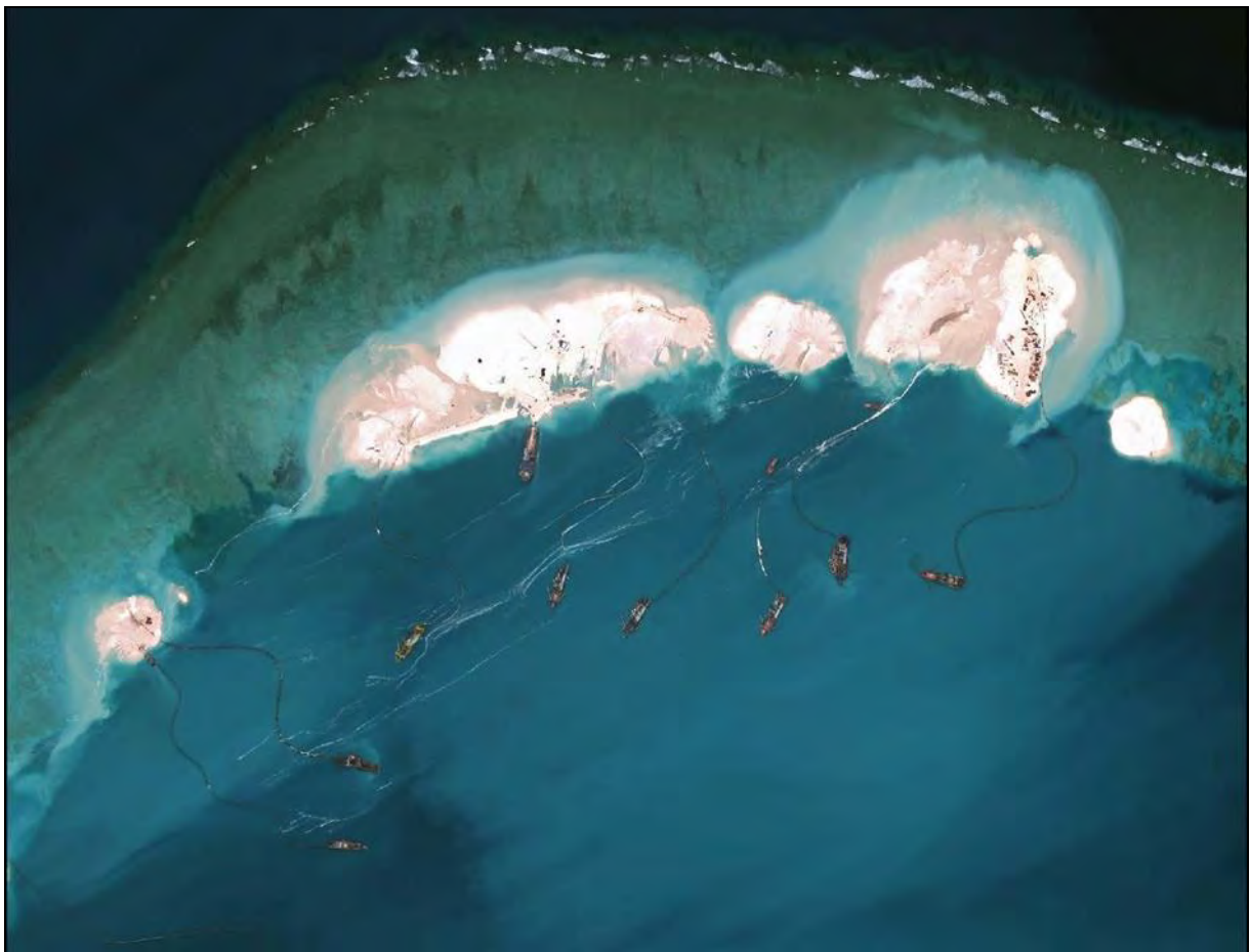
Figure 17: Dredgers at work at Mischief Reef (Annex 792)
